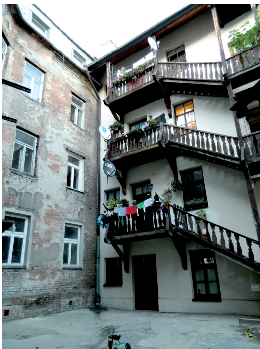
III. 1. Characteristic architecture of interblock spaces in the Old Town of Lublin – wooden galleries of annexes. Source: D. Chylińska (2012)
