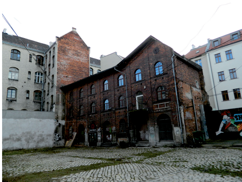
III. 6. Gable-end walls of houses in an unkempt backyard at Włodkowica Street show where no-longer-existing buildings used to stand. Original cobbles can be seen in the central part. Source: Chylińska (2013)
